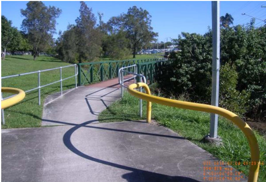
Waite Street Footbridge, looking downstream
