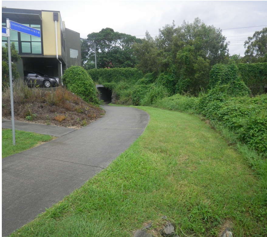
Cleveland Rail - Single bikeway culvert
