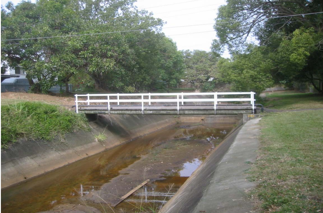
Sunshine Avenue / Barr Street Footbridge, looking upstream
