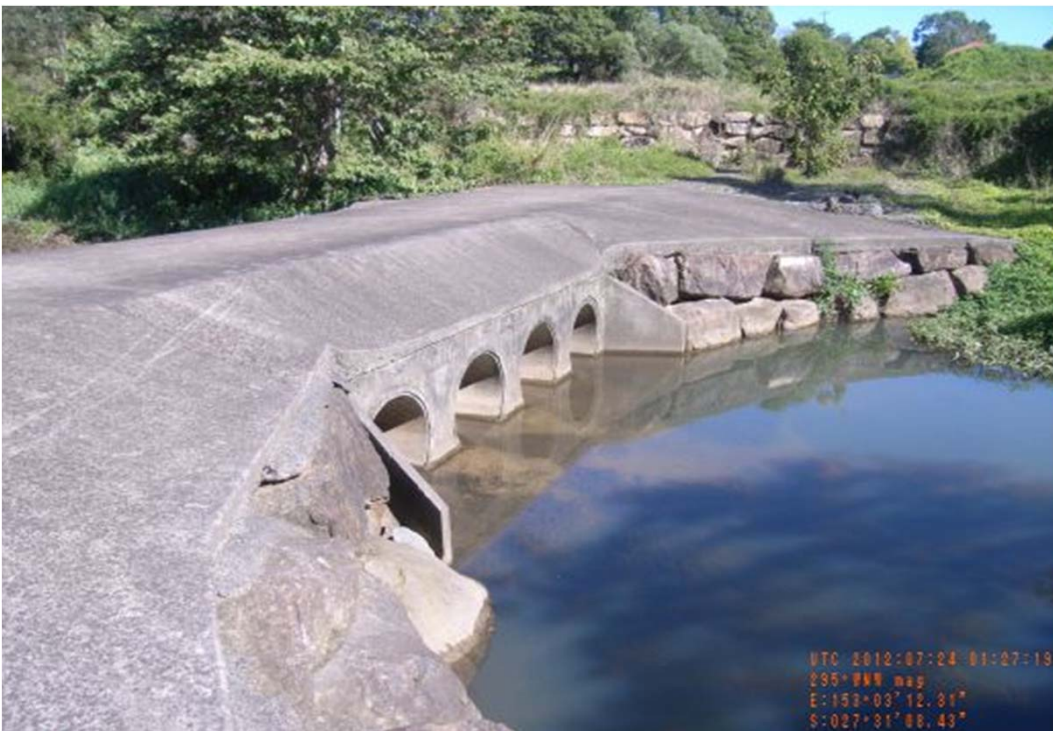
Birdwood Street, Development Causeway, looking upstream
