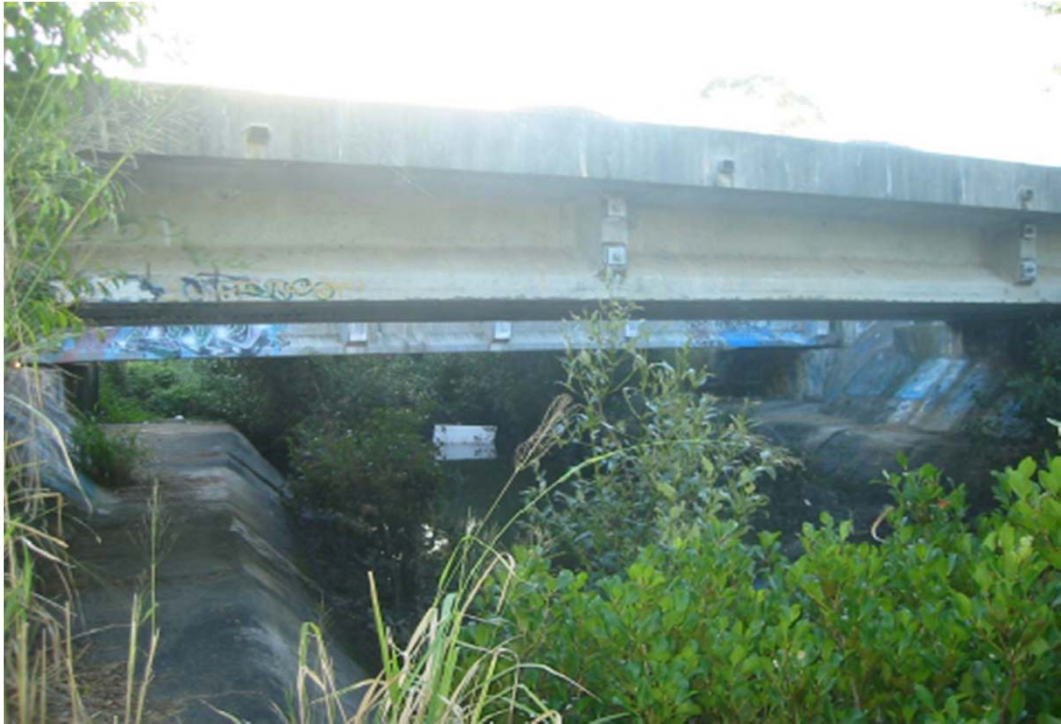
Cleveland Rail, looking downstream
