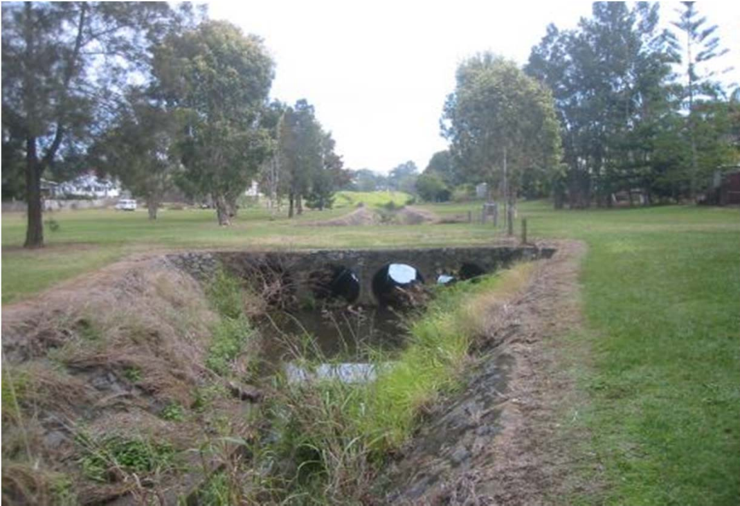
Maintenance Access, Joachim Street, looking downstream
