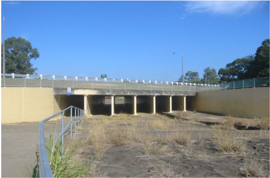
Ridge Street, looking upstream
