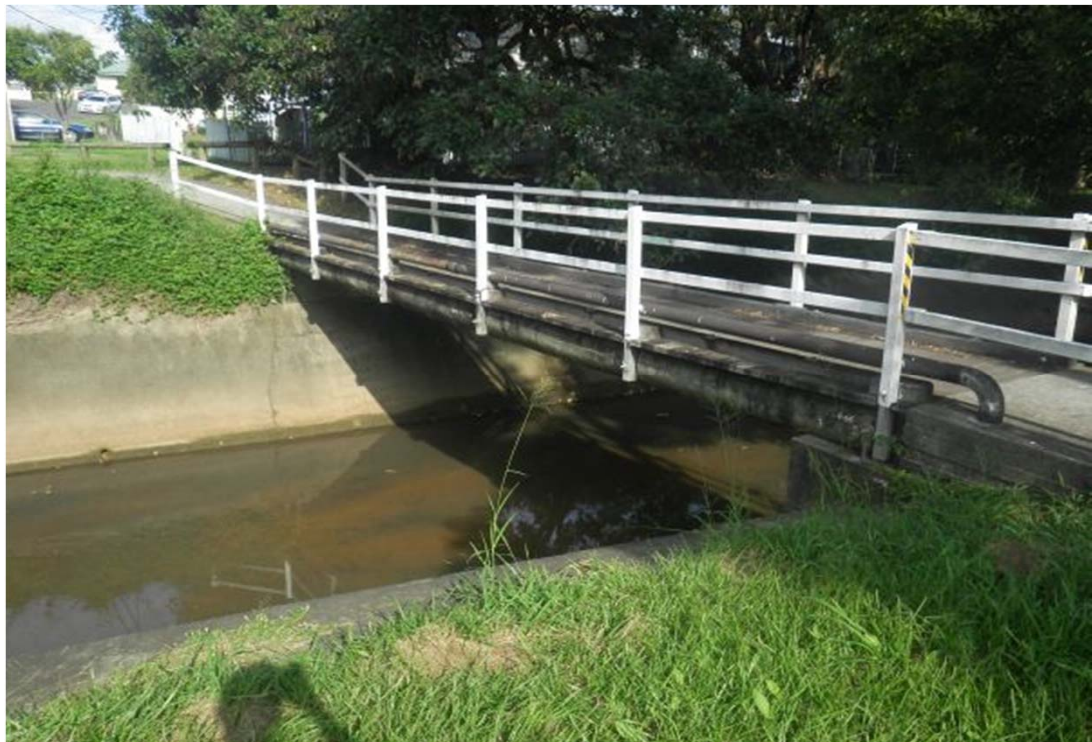
Sunshine Avenue / Barr Street Footbridge, looking upstream
