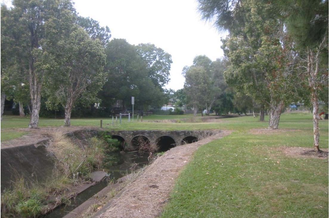
Maintenance Access, Joachim Street, looking upstream
