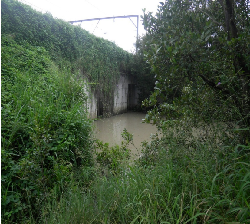
Cleveland Rail - Main set of culverts
