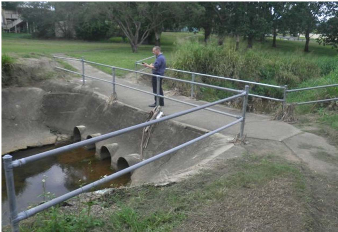
Glindemann Park Footbridge looking upstream
