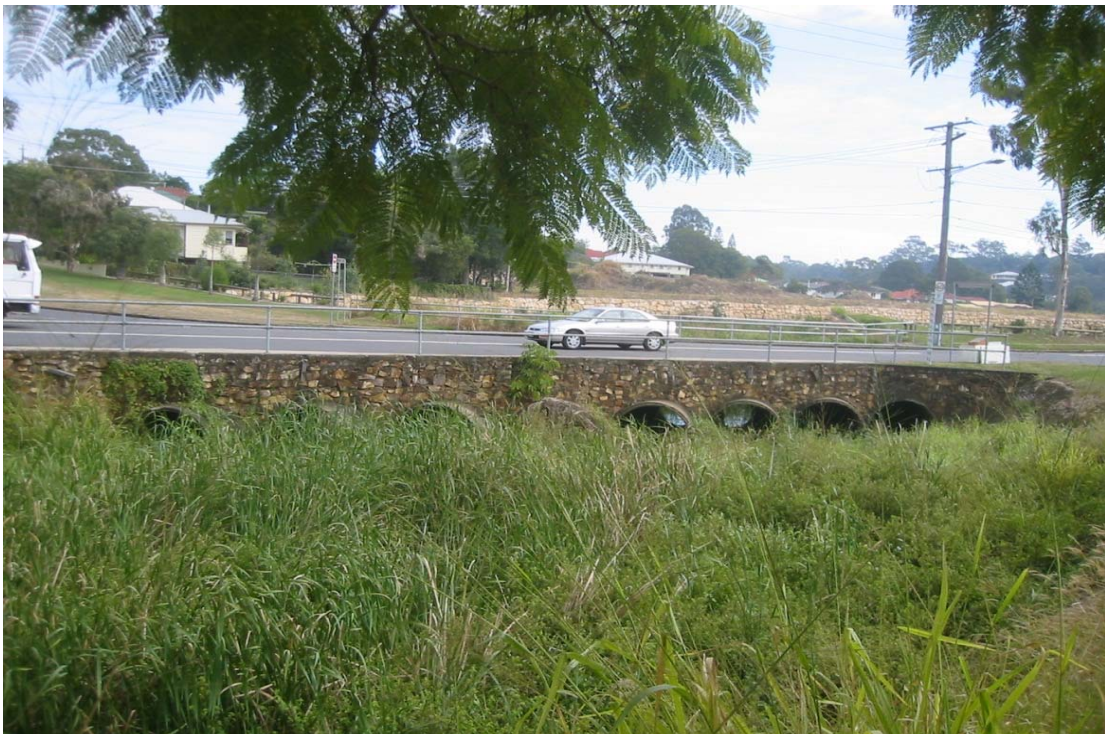
Birdwood Road, looking downstream
