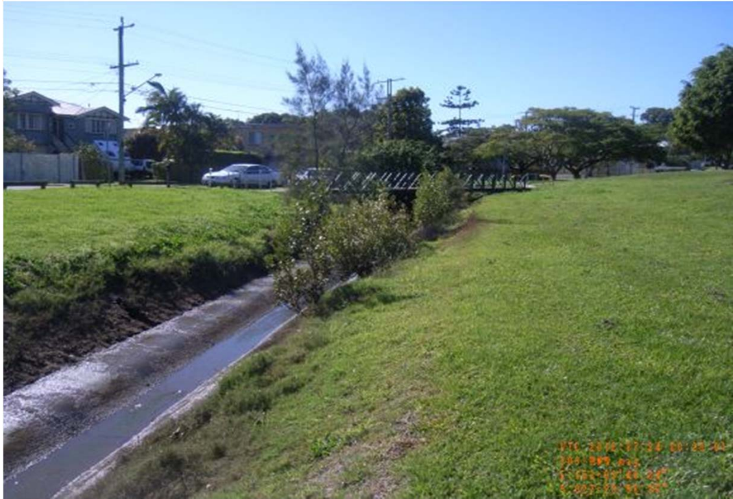
Waite Street Footbridge looking upstream
