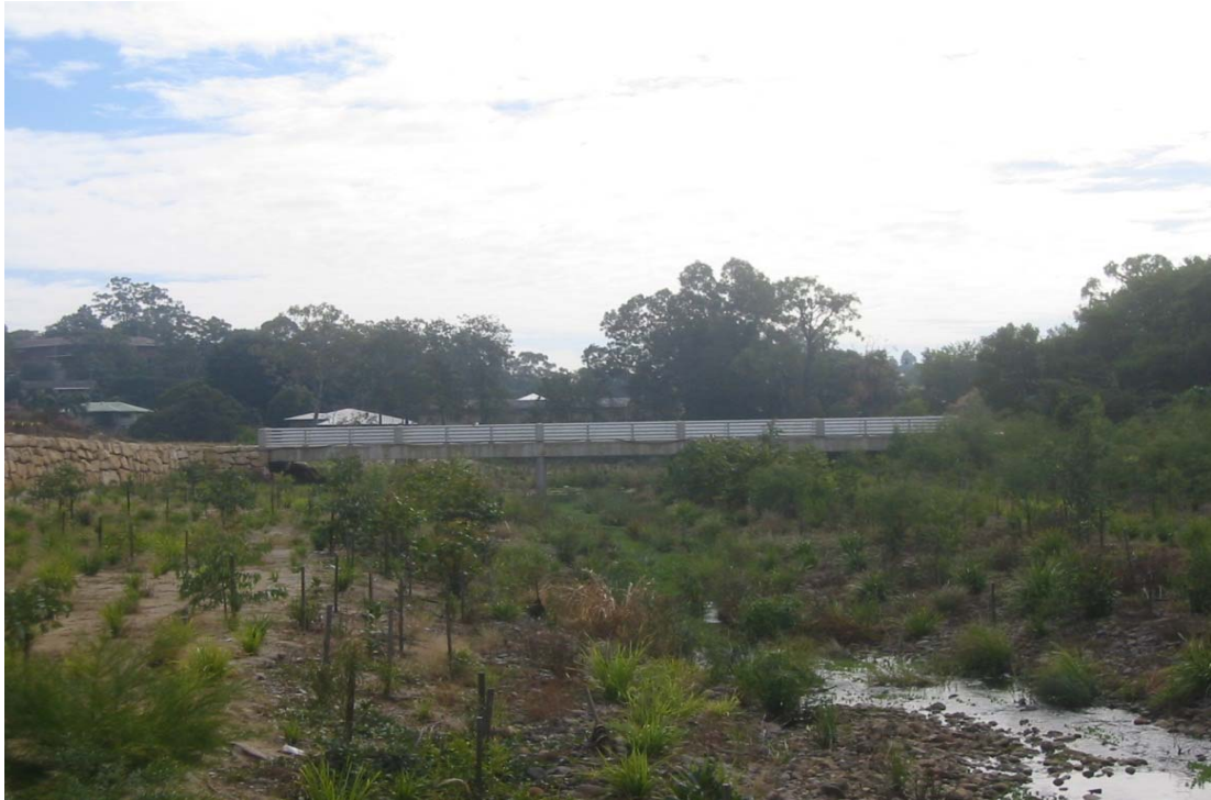
Birdwood Road, Development Bridge, looking downstream
